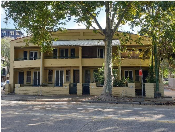
Figure 19. View to façade of 2A-2D Wentworth Park Road.
