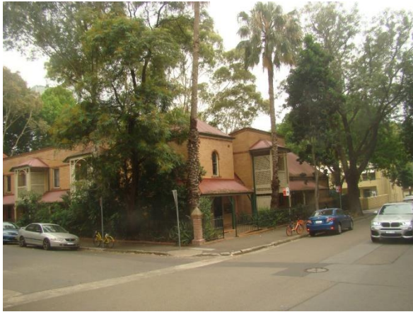
Figure 13. Overview of 17-31 Cowper Street.
