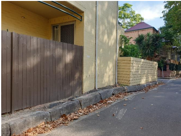
Figure 21. View of sandstone kerbing along Mitchell lane East.
