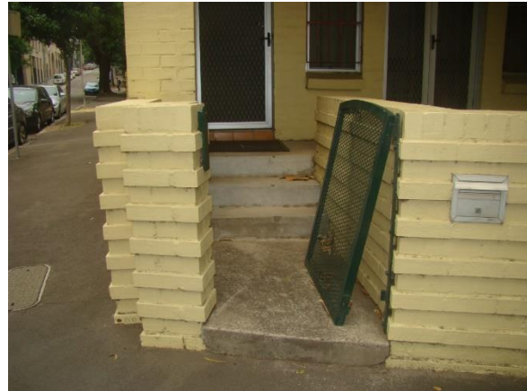
Figure 20. Entrance to 2A Wentworth Park Road.
