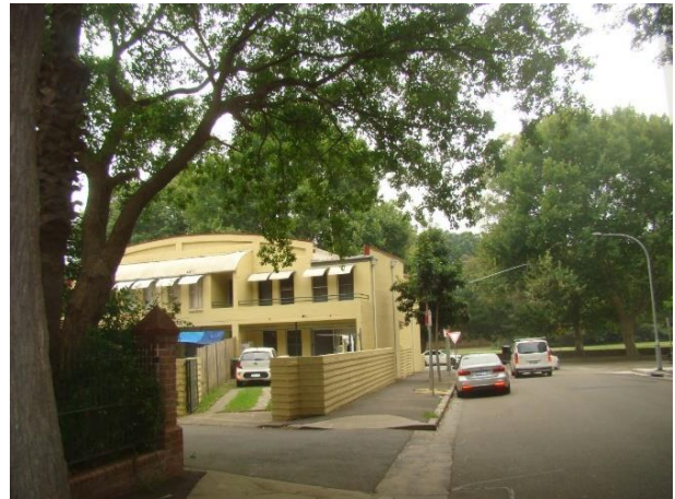
Figure 22. Overview of rear of 2A-2D Wentworth Park Road from Cowper Street.
