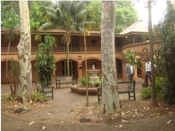
Figure 18. View to internal courtyard at 17-31 Cowper Street.
